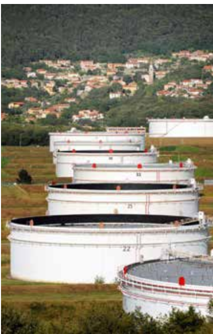
Transalpine Pipeline – Tanklager Triest.
